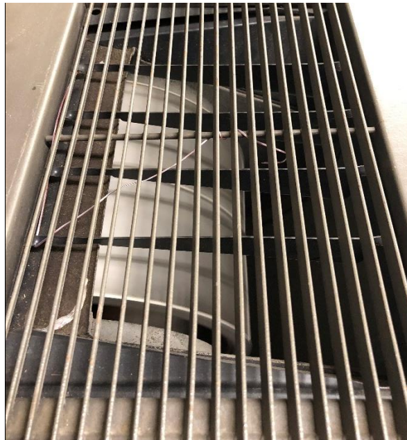
Figure 5: Air Supply Temperature Thermocouple Wire secured and hidden within UV grille
